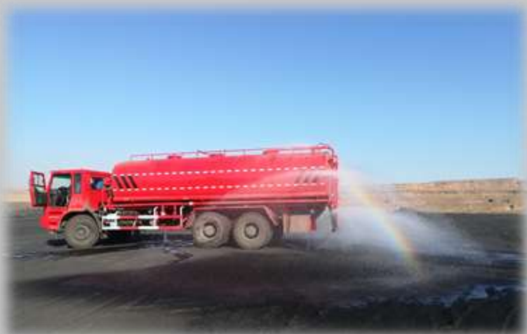
洒水车煤矿矿区施工。 Sprinkler coal mine construction.
